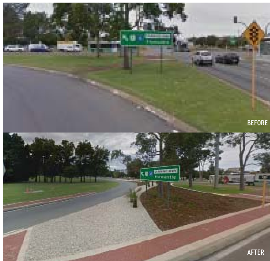
Image 9. Slip-road onto Canning Hwy from Albany Hwy
