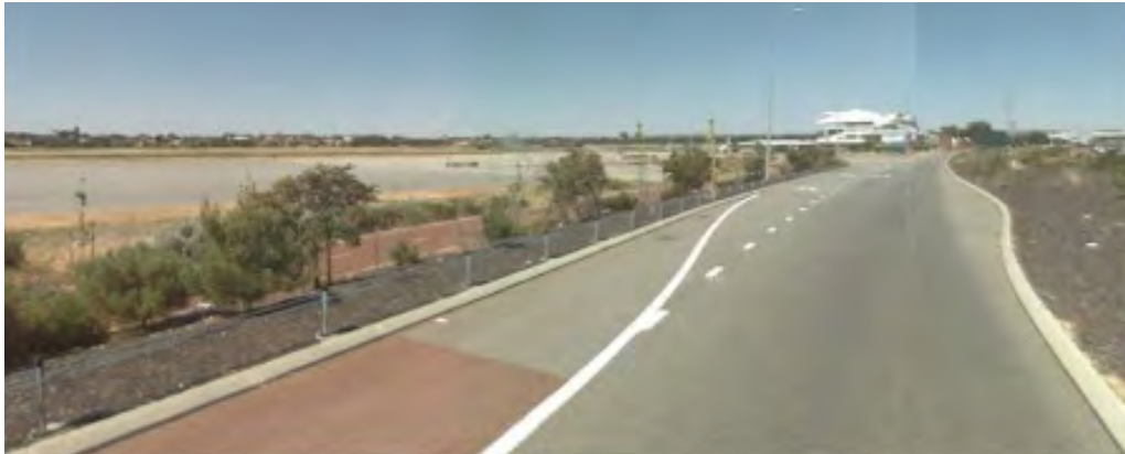
FIGURE 24: SITE APPROACH, VIEW FROM GRAHAM FARMER FREEWAY, ENTERING SITE
