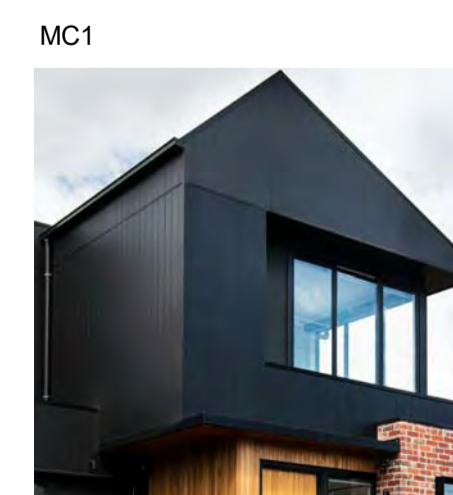
MC1 Black James Hardie Scyon cladding or similar to external wall / roof.
