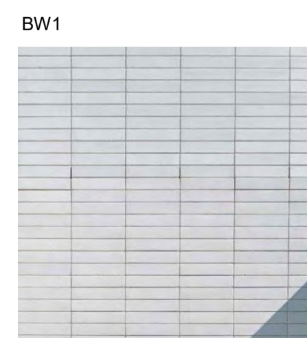
BW1 STACKBOND FACE BRICK; AUSTRAL MASONRY ENGINEERED STONE SMOOTH IN "HARVEST" 90W X 90H X 390L OR SIMILAR
