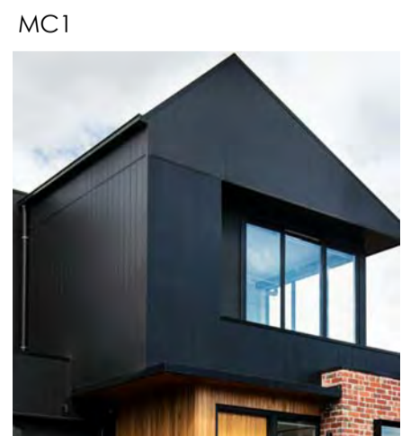
MC1 Black James Hardie Scyon cladding or similar to external wall / roof.
