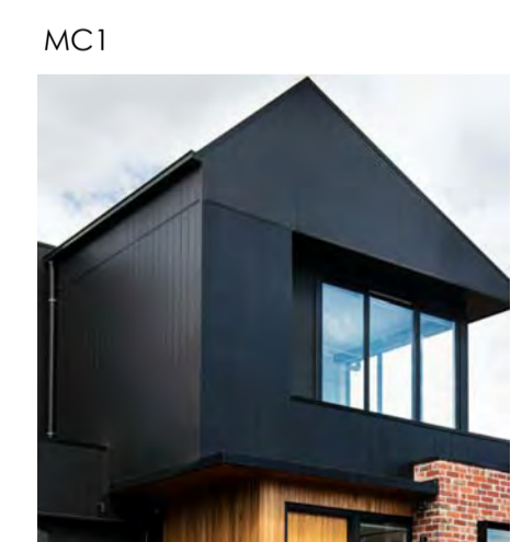
MC1 Black James Hardie Scyon cladding or similar to external wall / roof.
