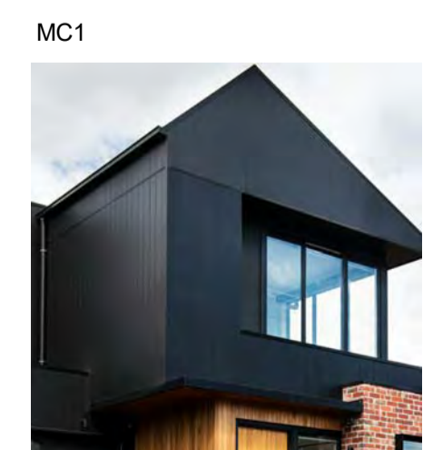
MC1 Black James Hardie Scyon cladding or similar to external wall / roof.
