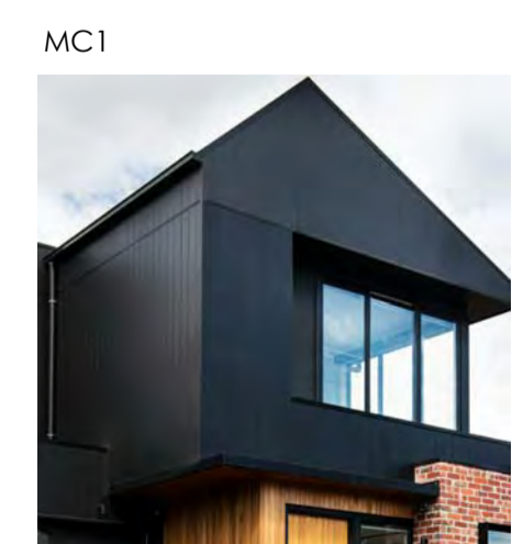
MC1 Black James Hardie Scyon cladding or similar to external wall / roof.
