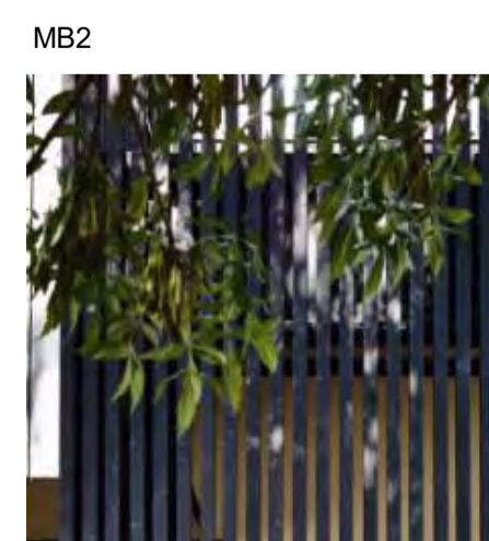
MB2 ARCHED TIMBER BATTEN SCREEN; 42X18MM DESIGN PINE PAINTED BLACK OR SIMILAR
