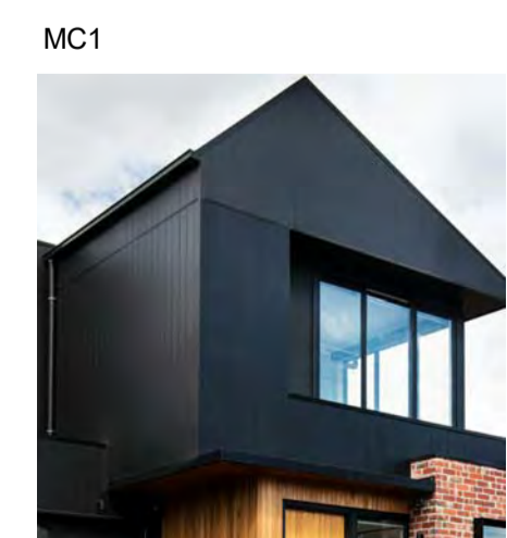
MC1 Black James Hardie Scyon cladding or similar to external wall / roof.
