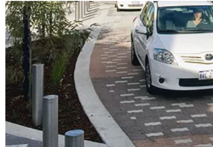
B3.3 Kerbs: In-situ Concrete (flush)
