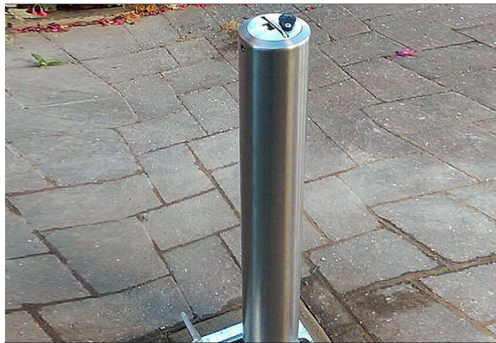
B3.5 Bollards: Automated Pop Up Bollards
