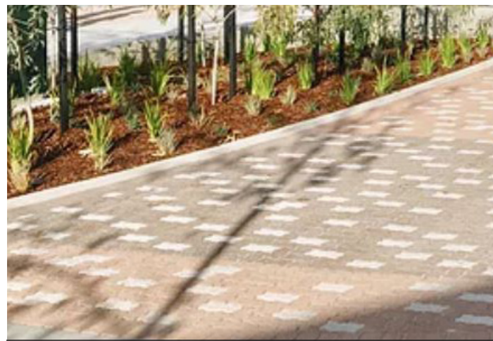
C3.1 Road Paving: Interlocking Road Paver
