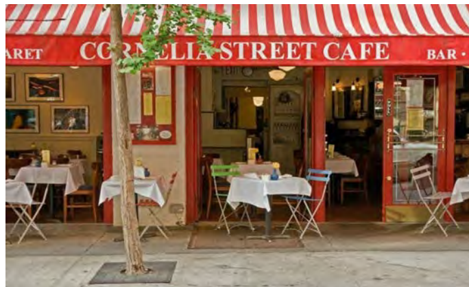
Figure 6. This is regarded as a good example of how street level retailing can enliven street activity during operating hours while still providing street character after hours. It succeeds because of its fine-grained detailing, materials, and colour and scale.
