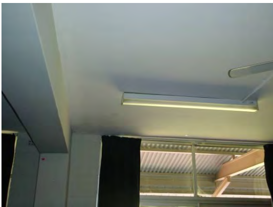
Figure 67 President's Lounge Toilet Window
