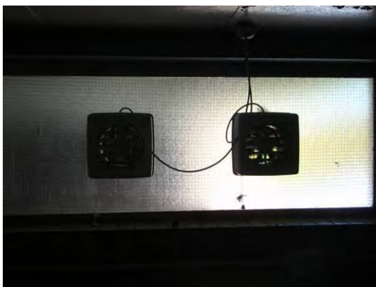
Figure 61 Perth Football Club 'Ice' Room Window
