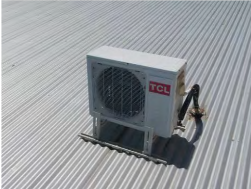
Figure 1 External Condenser
