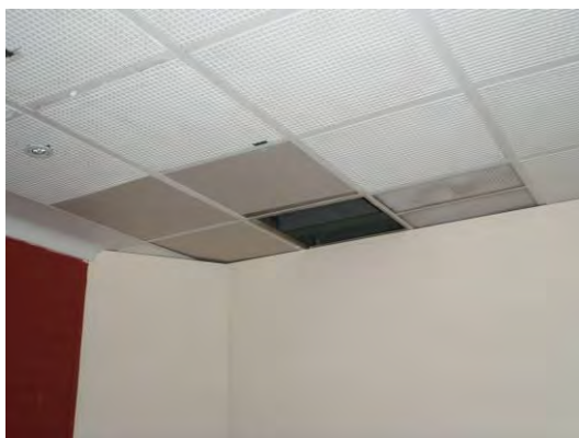
Figure 49 Back of Function Room Suspended Ceiling
