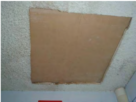
Figure 89 Office Area Roof Hatch
