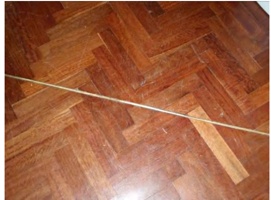
Figure 52 Function Room Wooden (Parquet) floor
