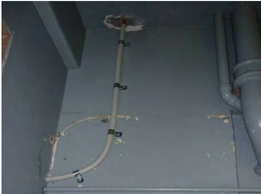
Figure 126 Work Unfinished in the Shower Room Opposite the Players Locker Room
