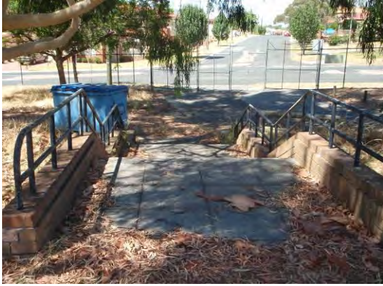
Figure 99 Entrance stair behind the Bar on the Hill
