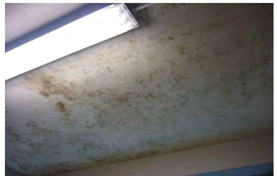
Figure 143 Water Leaking Stains in the Showers under the Bar
