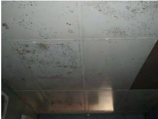
Figure 57 Perth Football Club 'Ice' Room Ceiling
