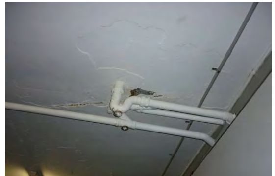
Figure 141 Spalled Concrete next to the Pipe under the Bar
