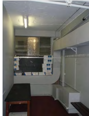
Figure 8 Redundant Ductwork
