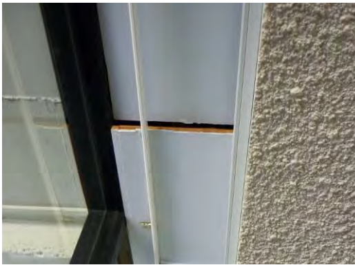
Figure 128 Movement in the Wood Ceiling in the Administration Office
