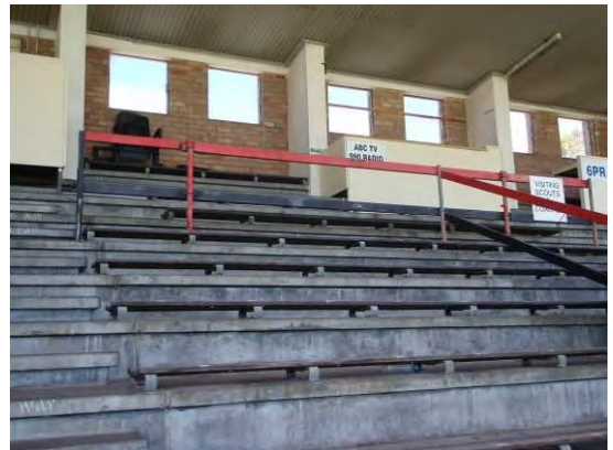
Figure 96 Grandstand Illustrating Makeshift Handrails
