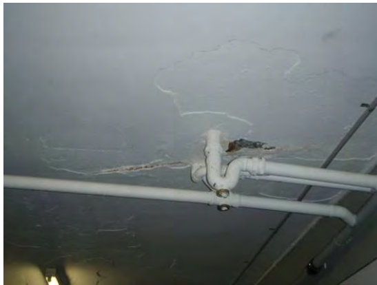
Figure 77 Visitors Changing Rooms Ceiling
