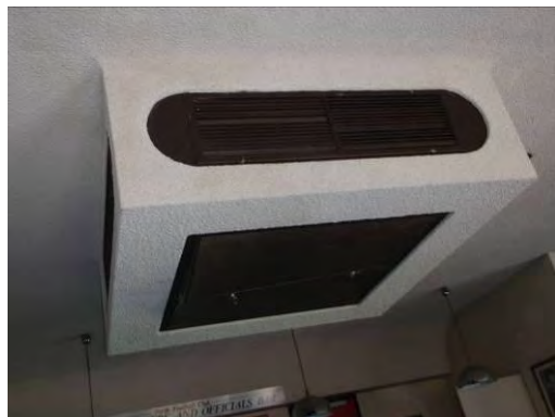
Figure 6 Redundant Evaporative (Internal) Air Handling Unit
