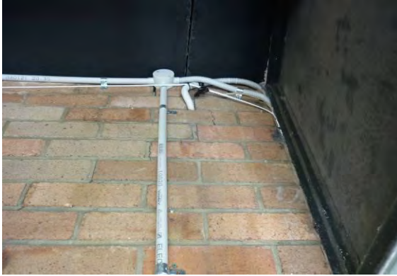
Figure 114 Crack in the Brickwork under Main Stand (West Side)
