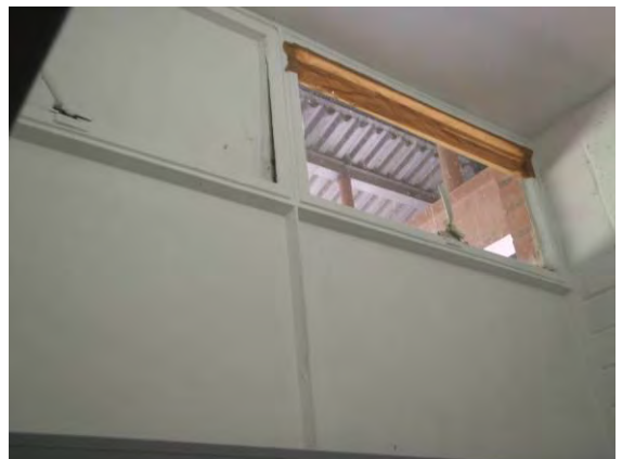
Figure 68 President's Lounge Toilet Window
