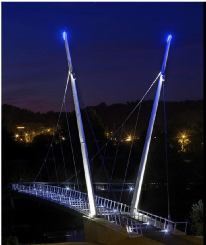
Figure 7: Reference image - Up lighting to Pylon
