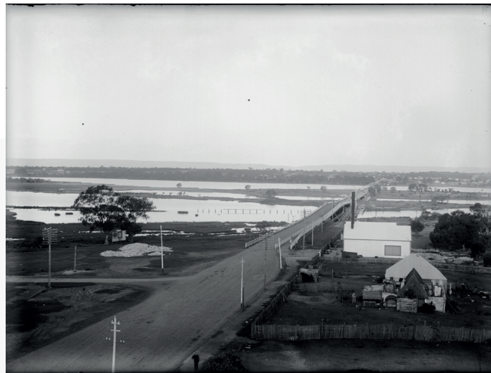
Figure 23. The second causeway, c. 1905. A tramway crossing is being constructed on the south side. (SLWA 006166PD)
