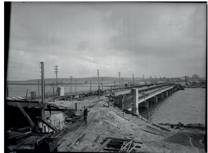
Figure 24. Today's causeway under construction in 1951. (SLWA 235184PD)
