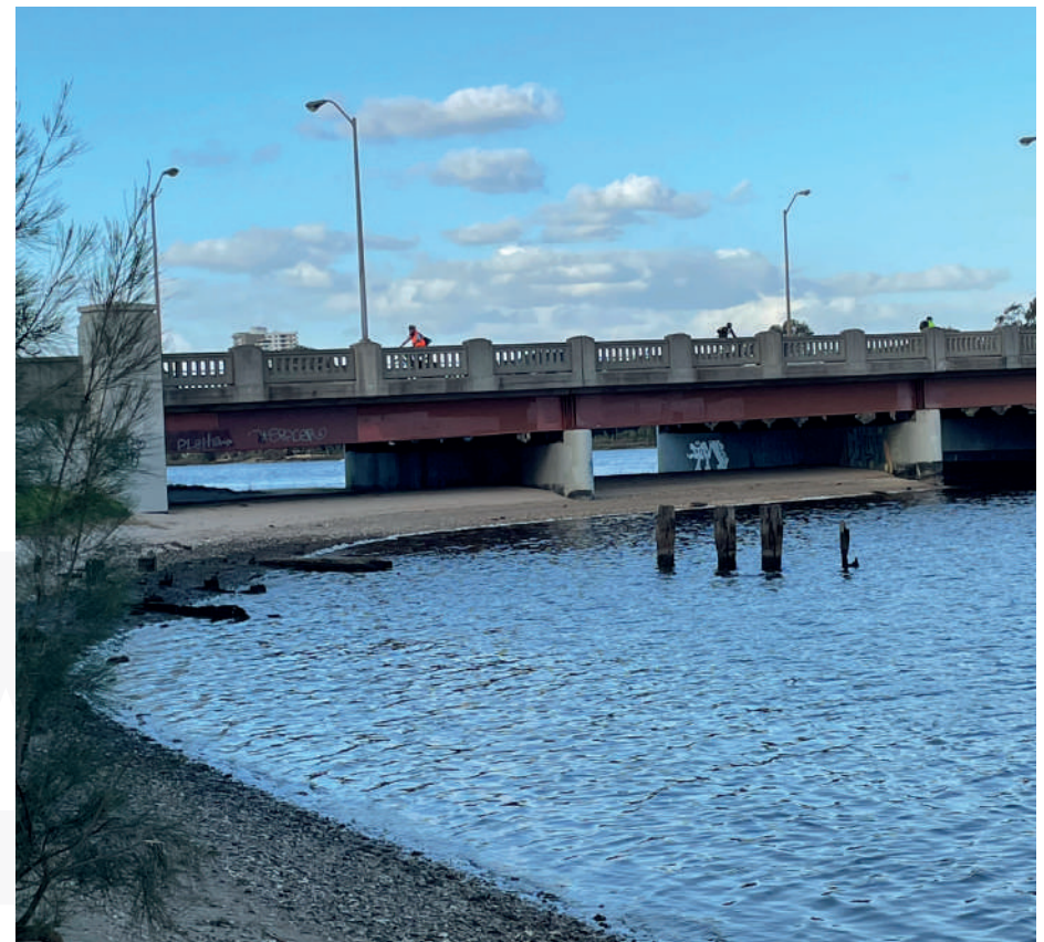
Figure 6. Eastern Causeway Bridge, with remnants of the second bridge in the foreground. (element 2021)
