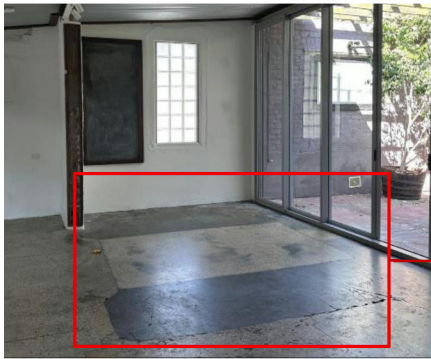
Image – Existing slab evidence of cracking and inadequate patching due to be replaced
