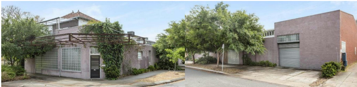
Image - Existing Façade – Geddes Street
