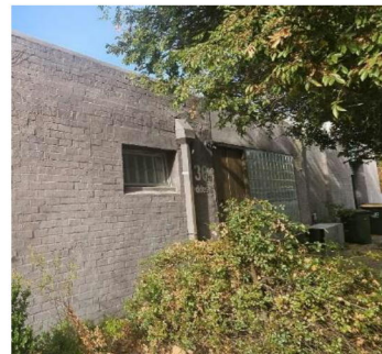
Images – Existing downpipes on the external Façade – Geddes Street and Washington St
