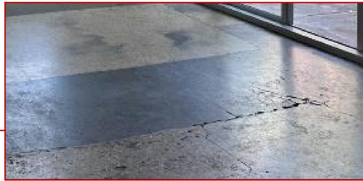
Image – Existing slab evidence of cracking and inadequate patching due to be replaced
