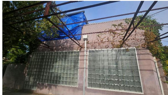
Image – Existing Façade – Geddes St
