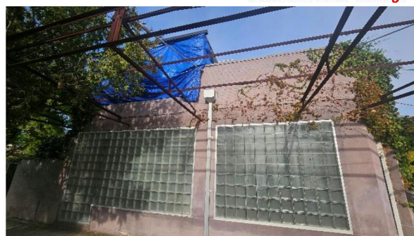
Images – Existing Façade tarps in place over existing balcony to protect from further weather damage – Geddes Street
