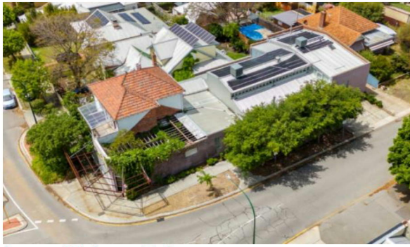
Image – Existing aerial view
