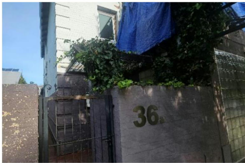
Image – Existing Façade – Geddes Street
