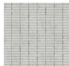
1c COMMON BWK IN STACKBOND WITH WHITE PAINT FINISH
