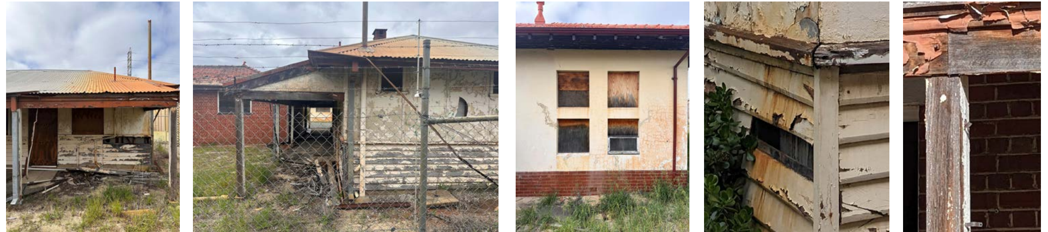
Weatherboard cladding with rendred wall above. Raw corrugated metal roofing. White painted timber details. Exposed jarrah structure.
