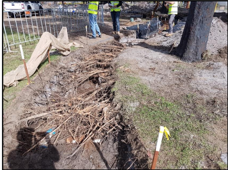
Figure 4. Example of vacuum excavations to uncover root mass – image supplied by Arbor Centre.
