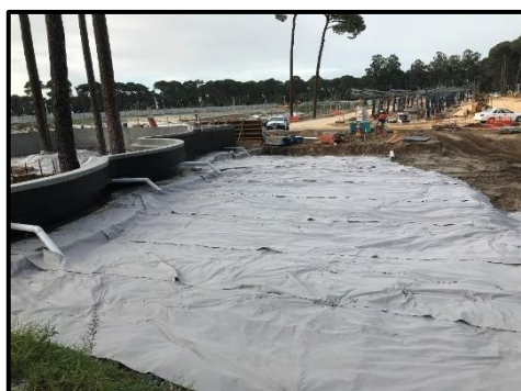
Figure 13. Example of Aeration Layer – Curtin Bus Exchange – Image source Arbor Centre
