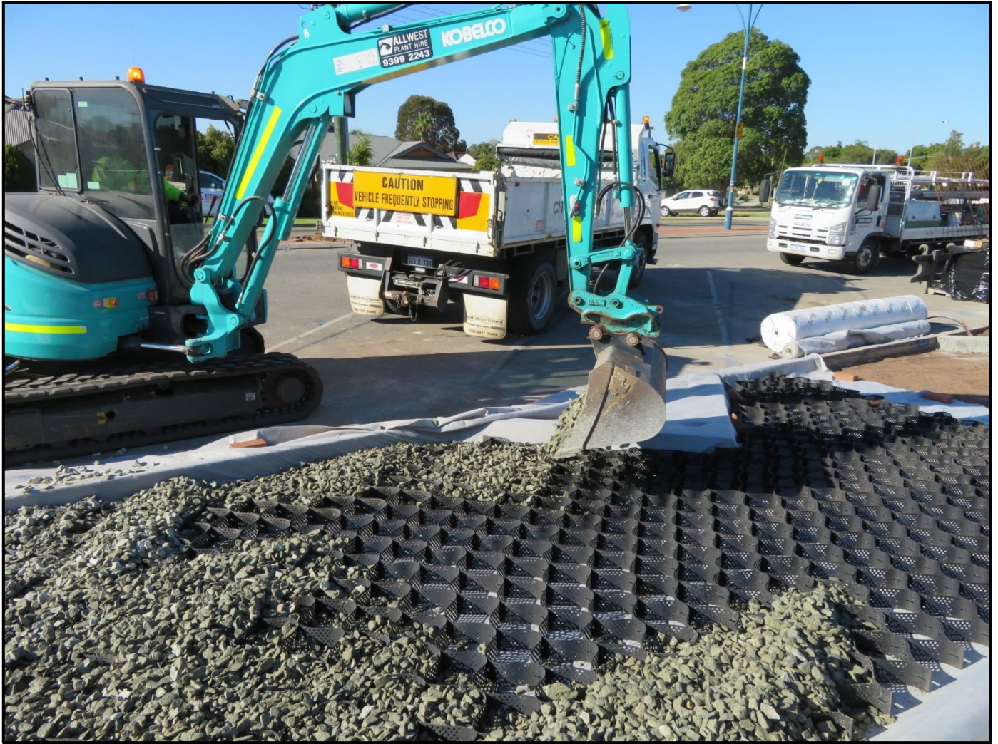
Figure 11. Example of GeoWeb product being installed within Epsom Avenue, Belmont – Image source City of Belmont (WA)
