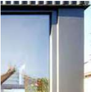
M8: Matte charcoal powdercoat glazing frames
