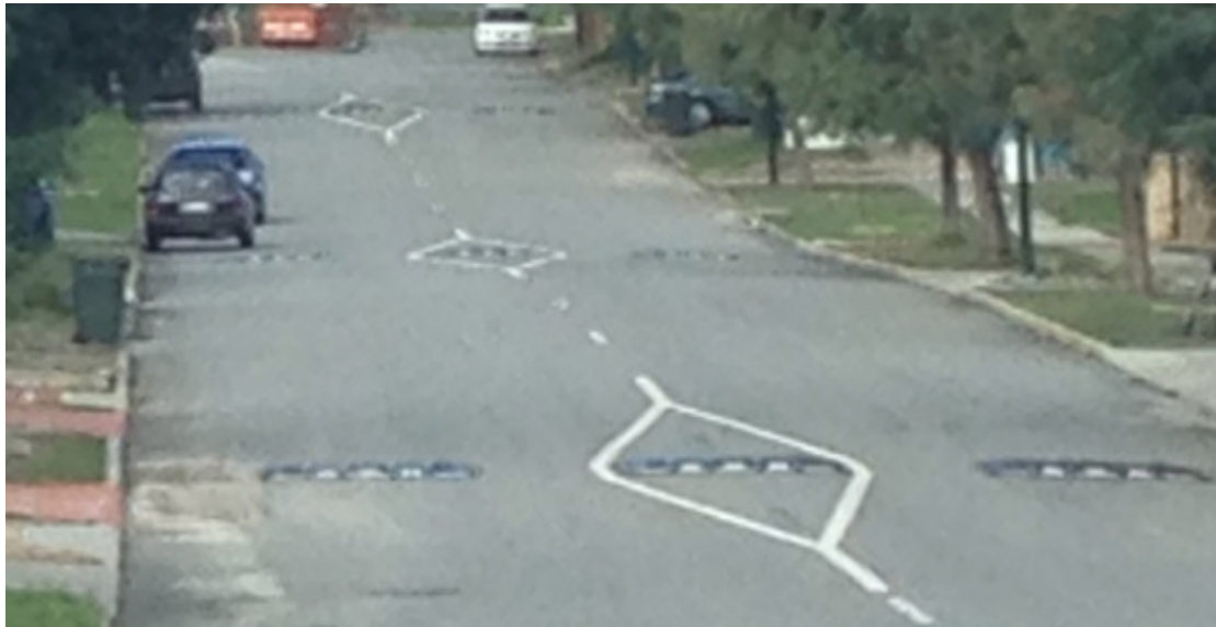
Figure B2.3 - Speed Cushions – as installed on Cornwall Street, Lathlain
