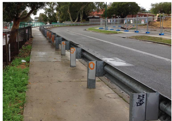
Figure 4.7 – Road Safety Barrier with Exposed Steel Posts
