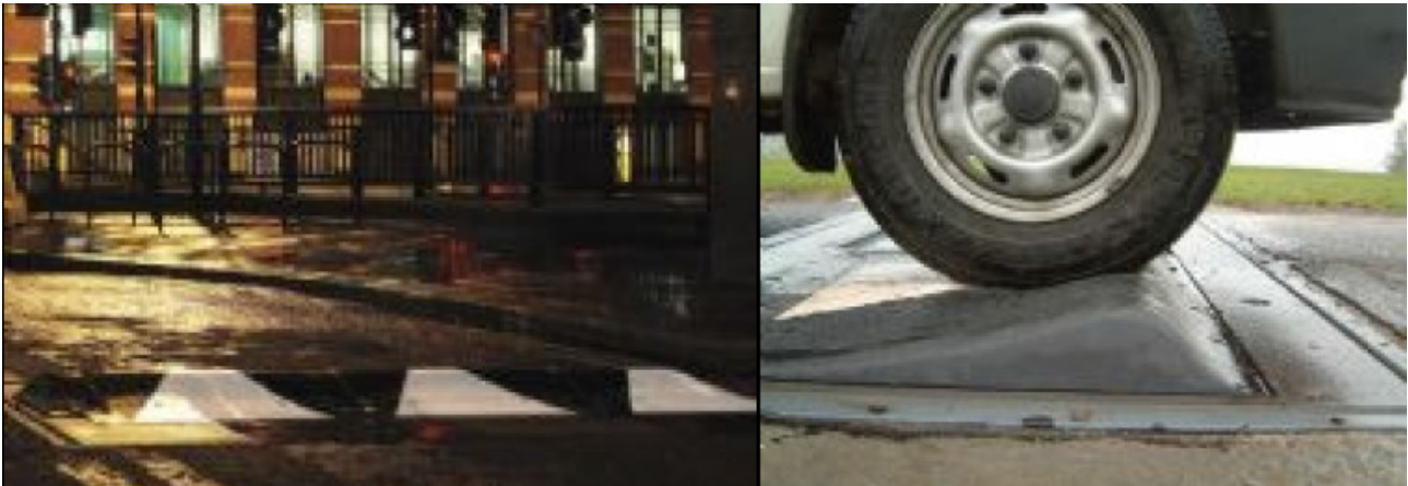
Figure B2.2 - Vehicle Responsive Speed Hump 27
