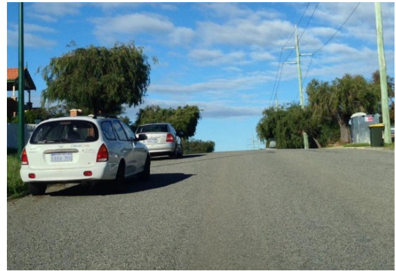
Figure 4.6 – Vertical Crest limiting Forward Visibility
