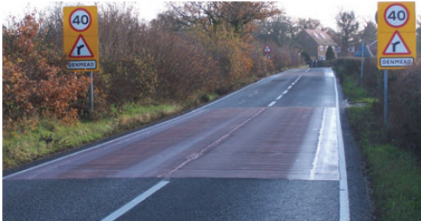
Recommended Profile for the Traffic Calming Surface
