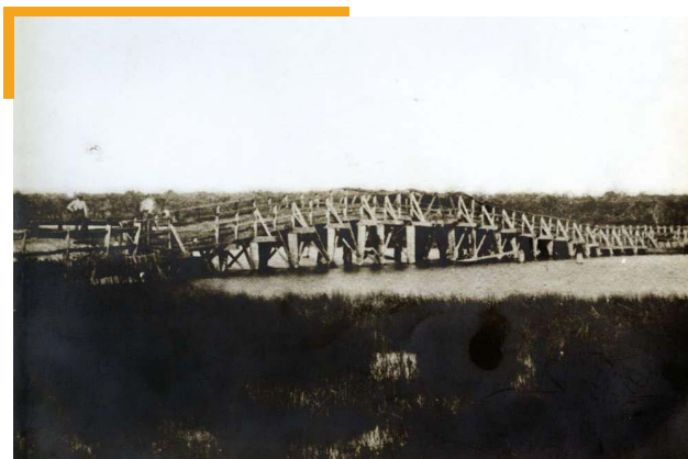
Original Causeway bridge built c1841 and destroyed by floods in 1862. Picture above taken in 1862 prior to its destruction.
