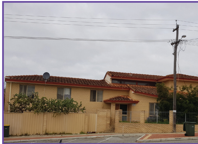
Lodging house and car park: 63 Etwell Street
