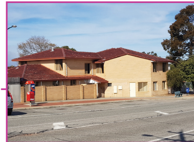
Lodging house and car park: 66 Etwell Street
