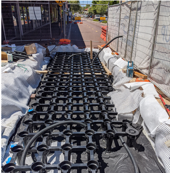
Structural Cells being installed below Albany Hwy paving.
