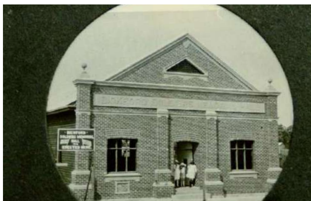
PH00005-03 Bickford Soldiers Memorial Hall, c. 1919 (nearly completed) Source: Historypin.org
