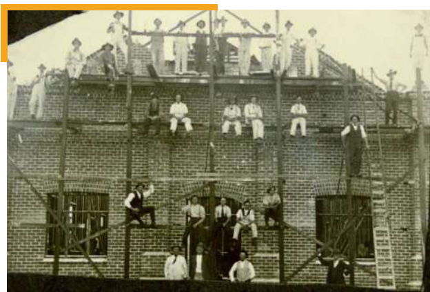
PH00005-05 Construction of the Bickford Soldiers Memorial Hall (PH40013)
