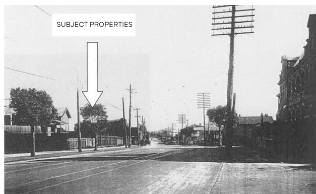
View of Albany Highway 1929
