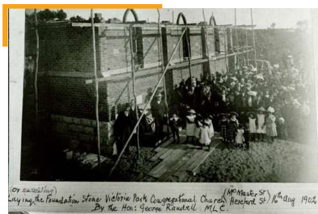
PH00026-01 Laying the foundation stone of the Victoria Park Congregational Church Unveiling of the Foundation Stone for the Victoria Park Congregational Church by Hon George Randell, MLC – 16 August 1902 (c of Perth)
