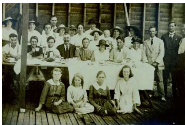
PH00003-01 Ladies Committee supply tea to building volunteers of the Bickford Soldiers Memorial Hall Source: Historypin.org
