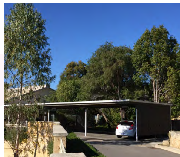
Figure 64: Existing Open Carport Parking
