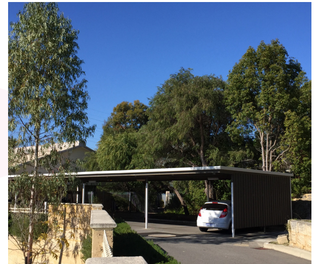
Figure 64: Existing Open Carport Parking
