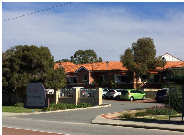
Figure 17b : Annesley Entry to Hill View Terrace
