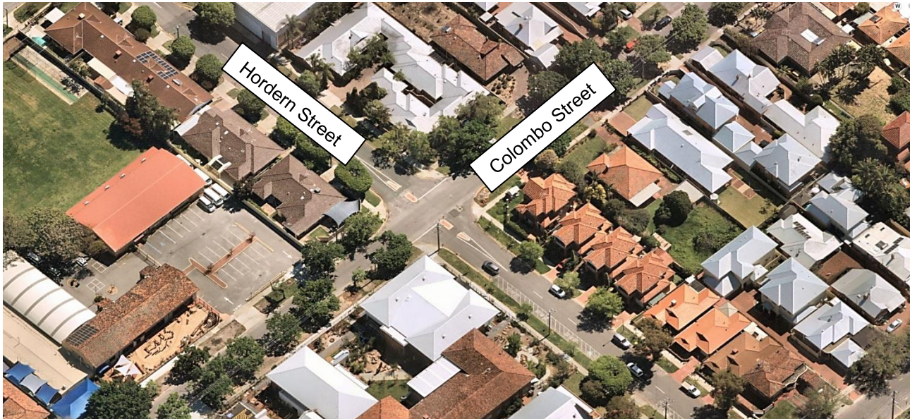
Figure 3-4 Hordern Street/Colombo Street Intersection
