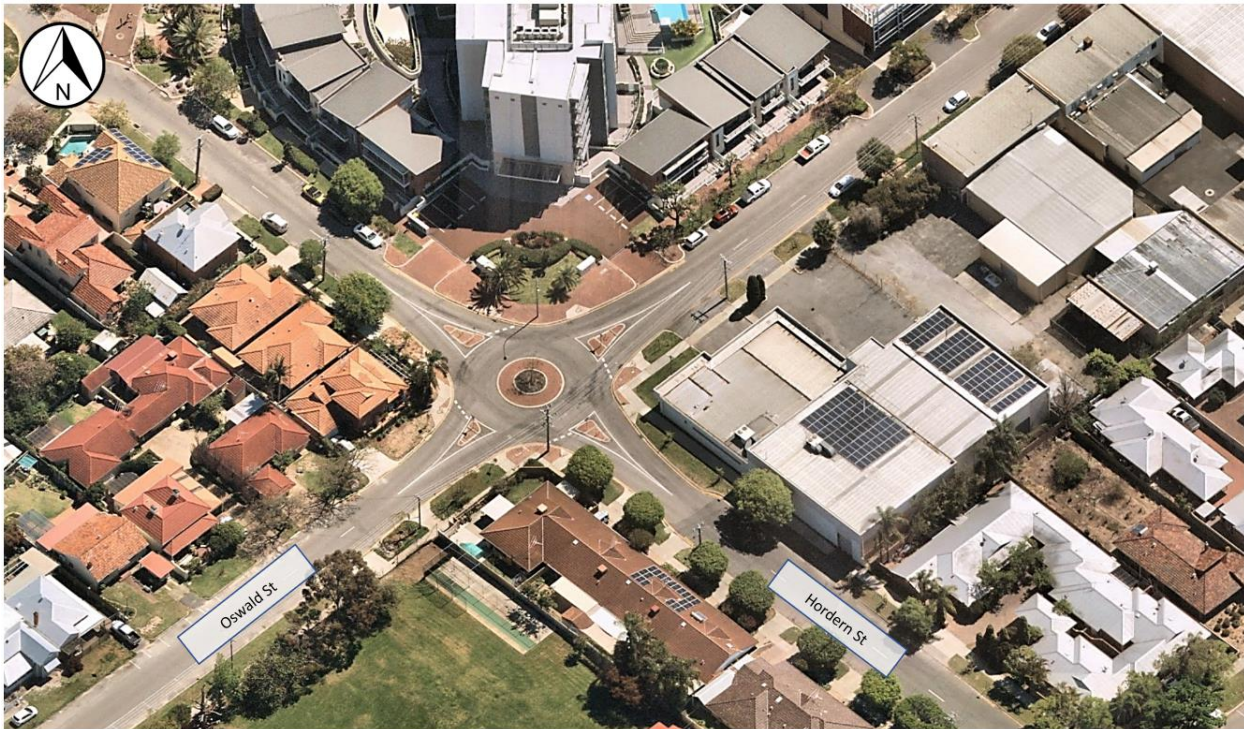
Figure 3.4 - Oswald Street/Hordern Street Intersection
