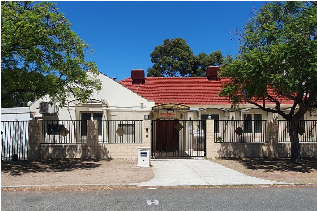
Above photo: showing front / pedestrian entry of church from Gerard Street
