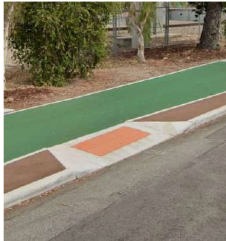
Align cross connectors with existing pram ramps
