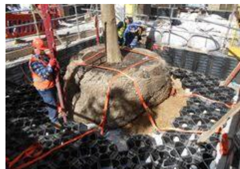
A Tree being planted with root cells around it, the pavement is then installed around the tree, over the cells
