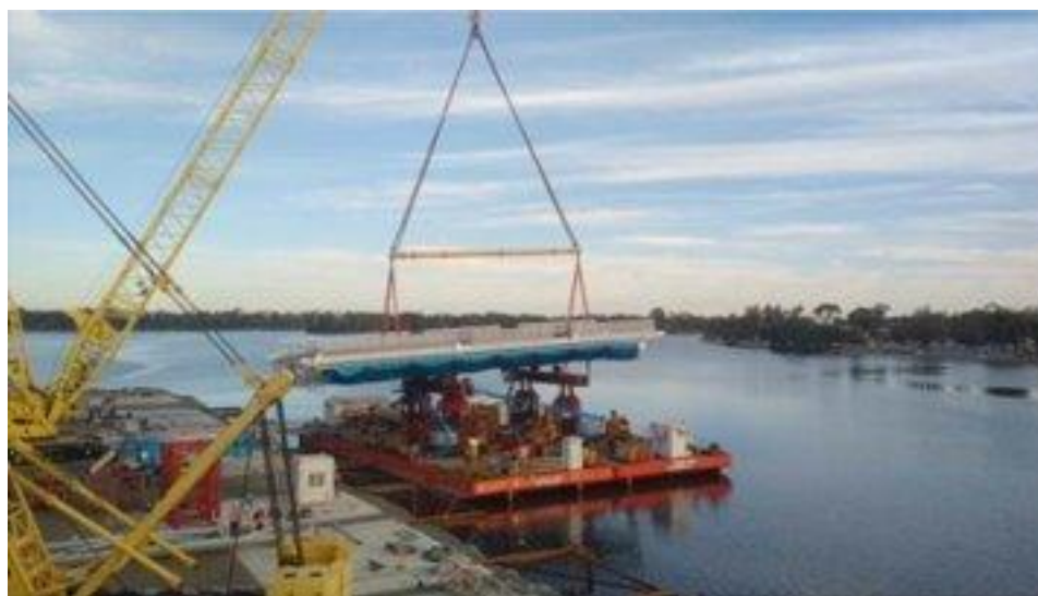
Figure 39: Bridge Segment Loaded onto Barge
