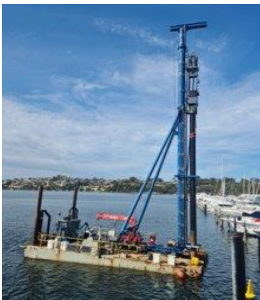
Figure 15: Typical Piling Barge Set-up
