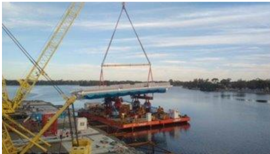
Figure 41: Bridge Segment Loaded onto Barge
