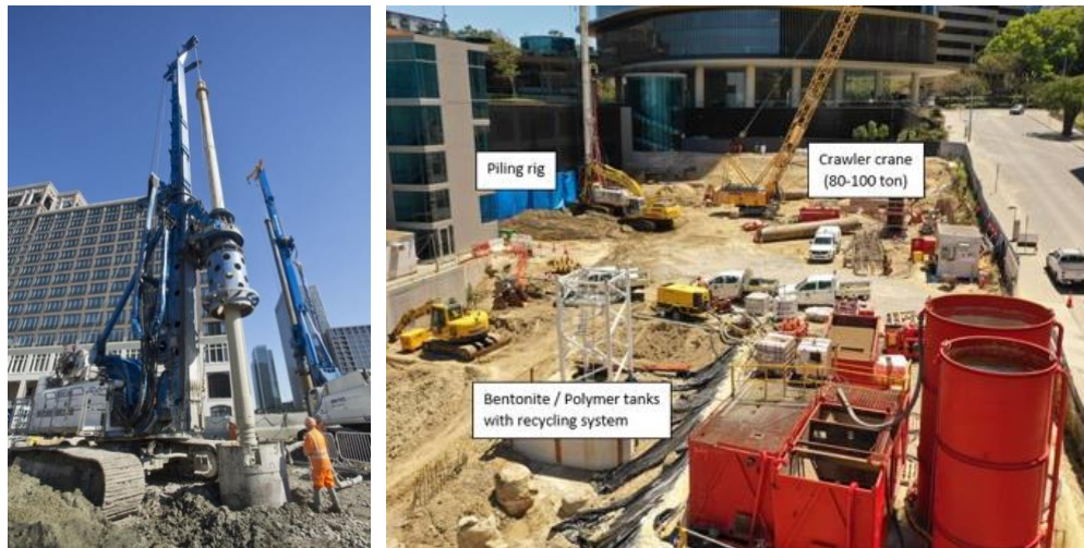
Figure 9: Typical Bored Piling Set-up
