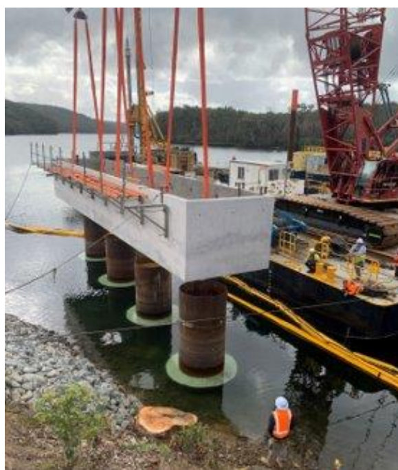
Figure 18: Typical Pile Cap Shell Installation
