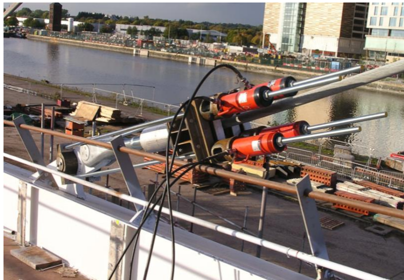
Figure 45: Typical Stay Cable Tensioning Device
