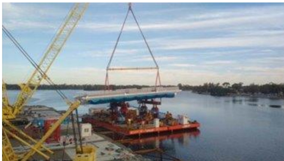
Figure 37: Bridge Segment Loaded onto Barge
