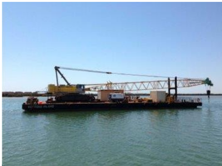
Figure 17: Crane Barge to Lift Portal Frames
