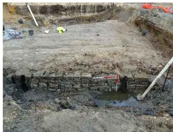
Plate 12. A section of dressed limestone wall of the Barrack Street Jetty
