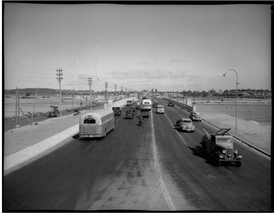
Figure 33. 1953 44 Causeway Bridge III with Causeway Bridge II on the left being demolished (slwa_b3416445_1)
