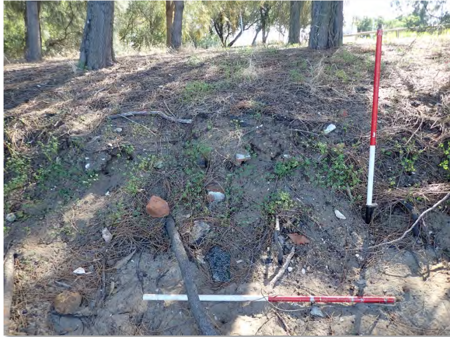
Plate 5. View north of southern bank of Heirisson Island behind remnants of Causeway Bridge II, showing rubble eroding out of bank
