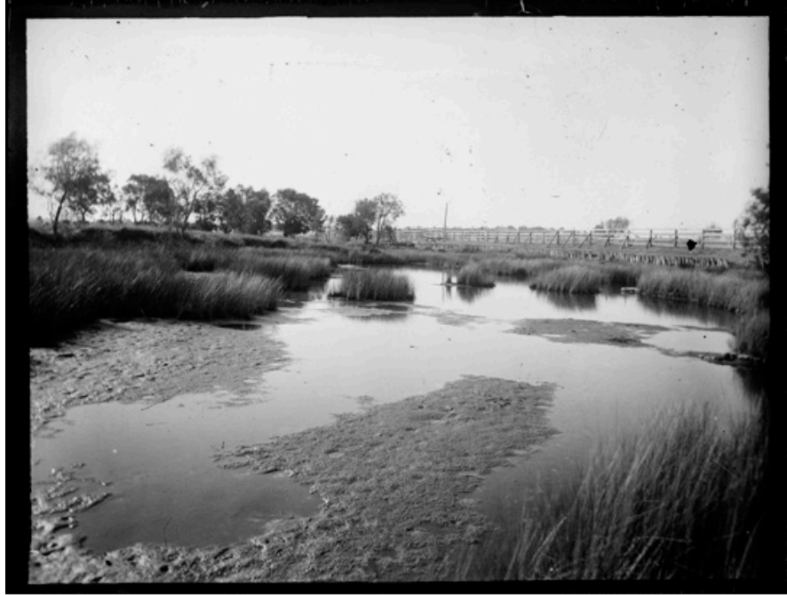
Figure 14. 1890s view of Causeway Bridge II and the mudflats (slwa 230443PD)
