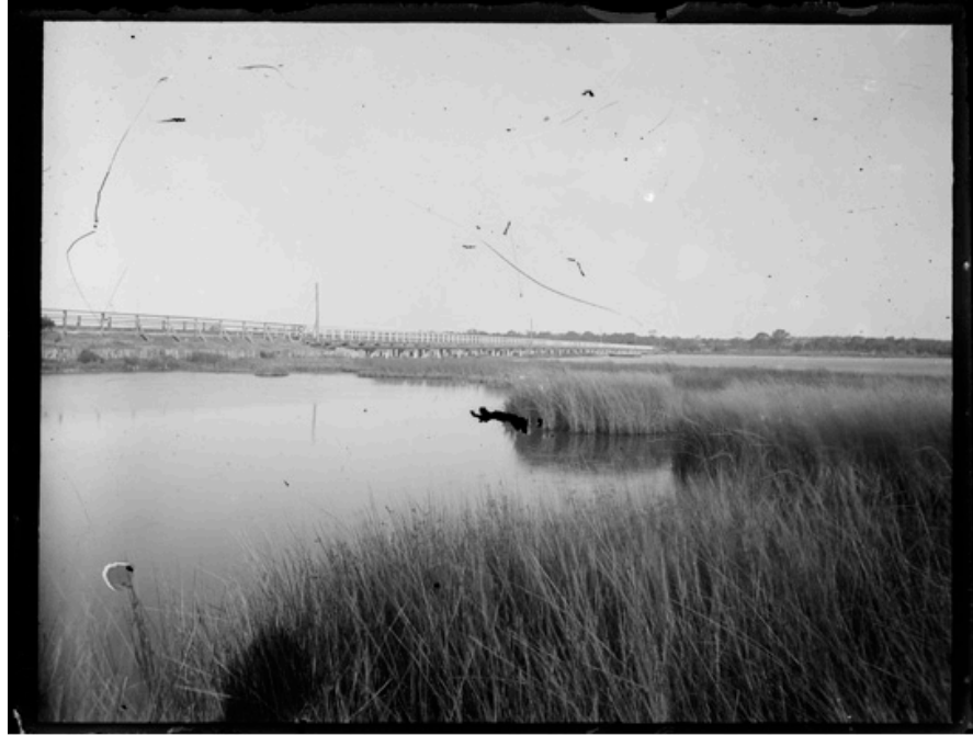
Figure 16. 1890s view of Causeway Bridge II and the mudflats (slwa 230445PD)
