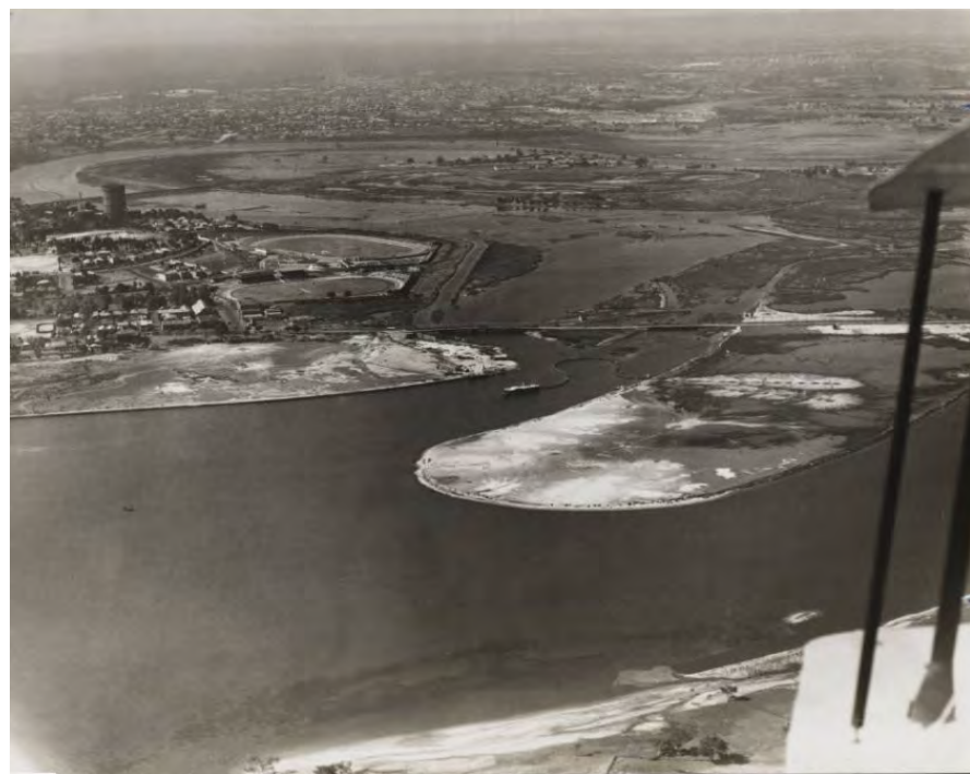
Figure 27. 1939 aerial view north of the Causeway and Heirisson Island (slwa_b6333109_3)
