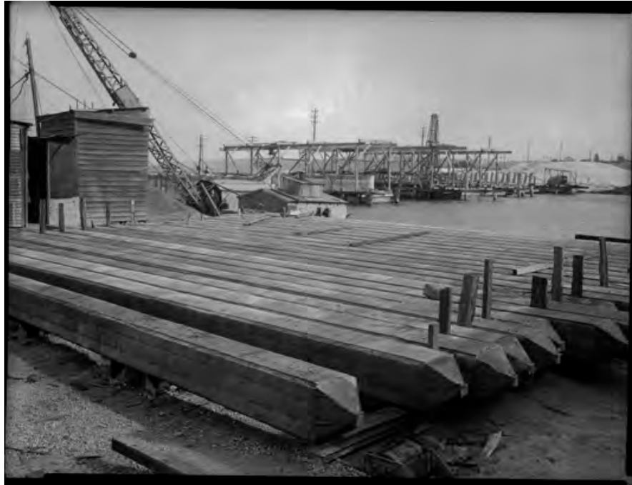
Figure 31. 1951 concrete piles for Causeway Bridge III (slwa 235,185PD)
