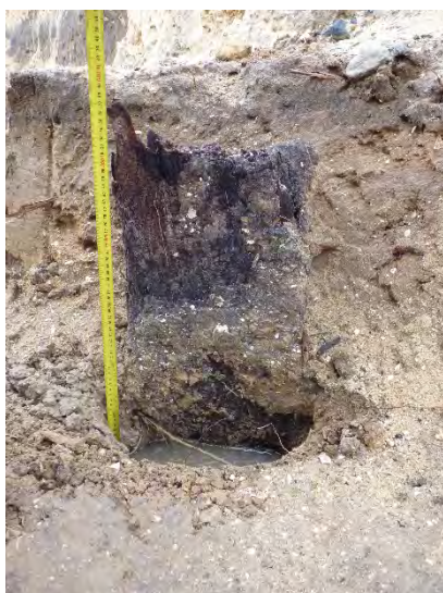
Plate 25. Jarrah timber piles found within reclaimed section of Perth Foreshore
