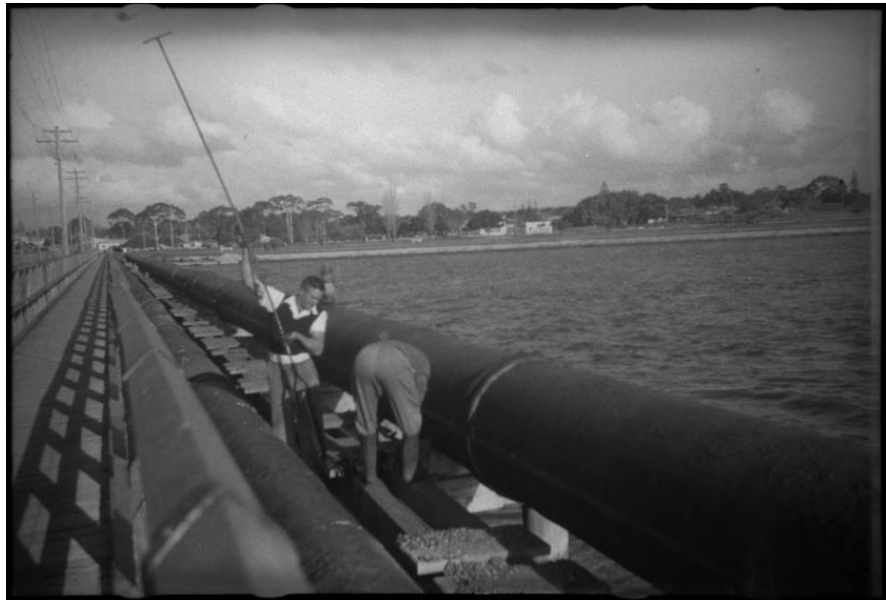
Figure 29. 1950s water pipeline beside the Causeway Bridge II (slwa_b6058474_1)
