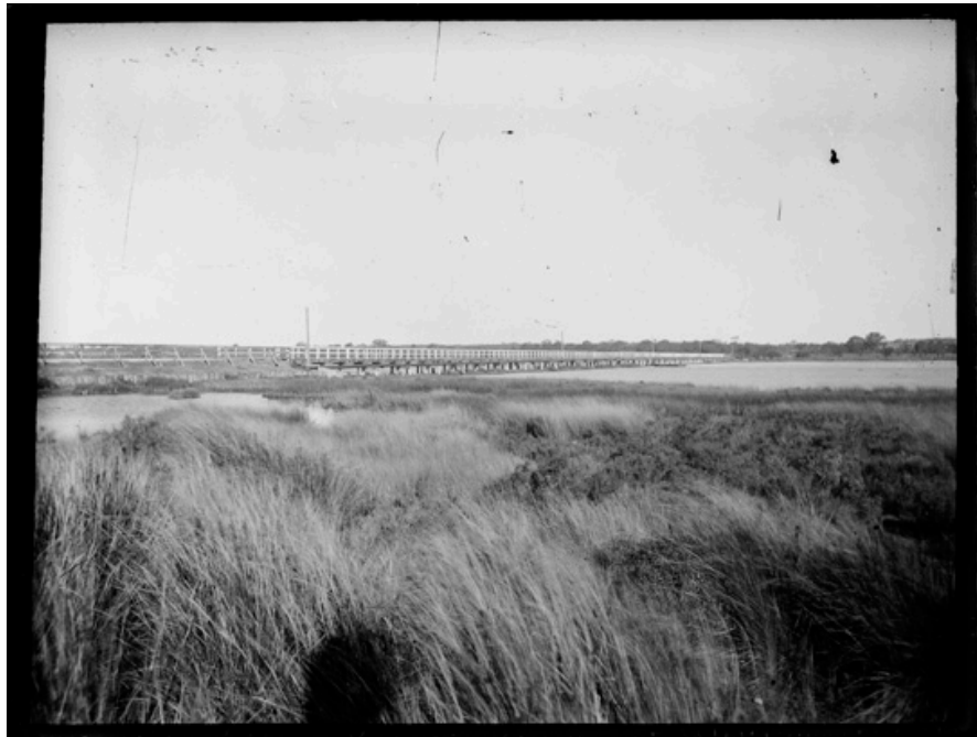
Figure 15. 1890s view of Causeway Bridge II and the mudflats (slwa 230444PD)
