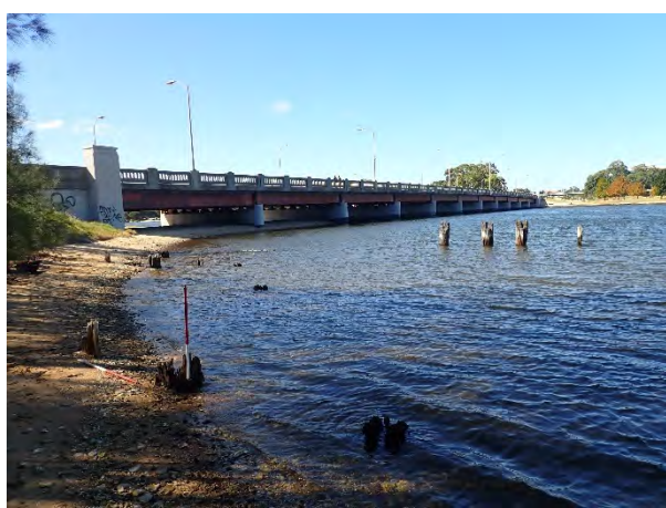
Plate 25. Jarrah timber piles found within reclaimed section of Perth Foreshore
