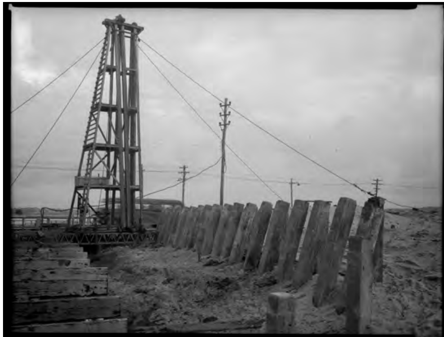
Figure 32. 1951 view of construction in progress for Causeway Bridge III (slwa 235,186PD)
