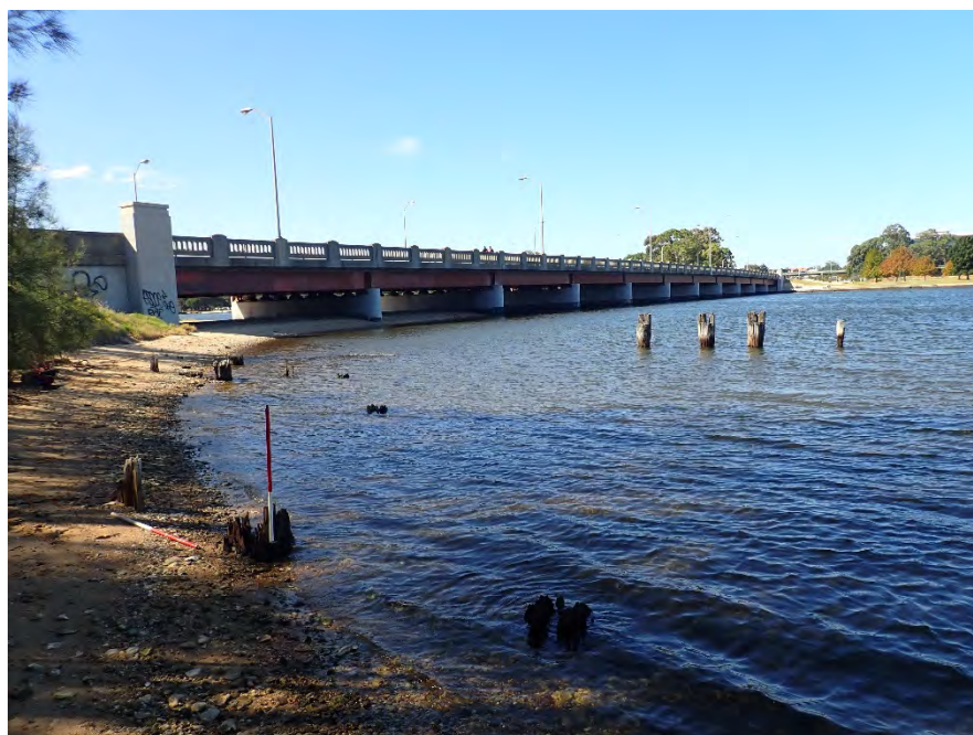
Plate 1. View East of timber piles and present Causeway Bridge (III)
