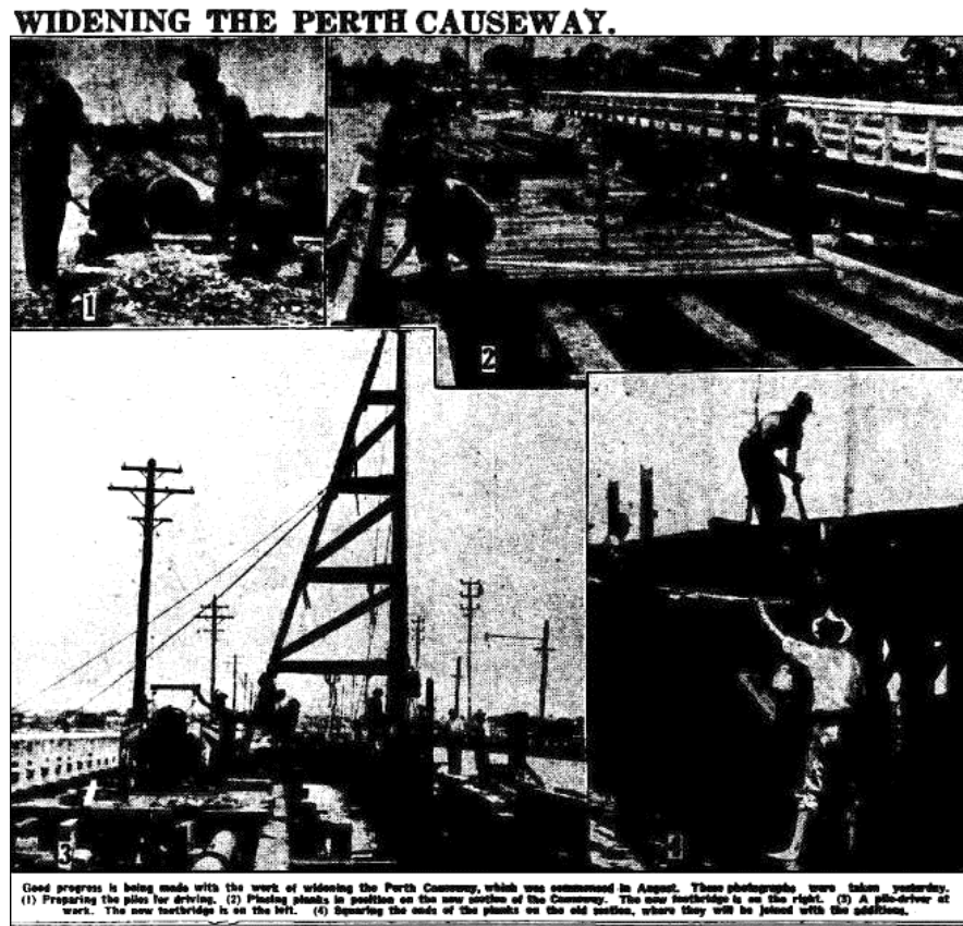
Figure 26. 1932 Causeway Bridge II widening works underway 42
