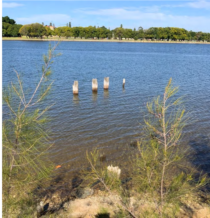
Plate 2. View southeast with large remnant timber piles in river and poorly preserved piles in foreground
