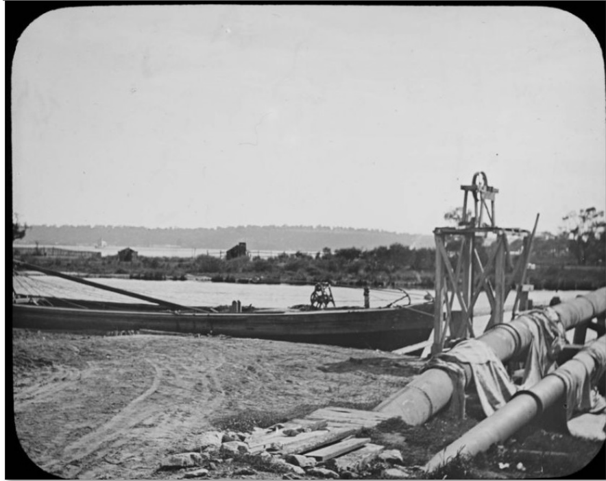
Figure 20. 1906-1907 pipes over the Causeway, with buildings present on Point Fraser in mid-ground (slwa_b2948373_21)
