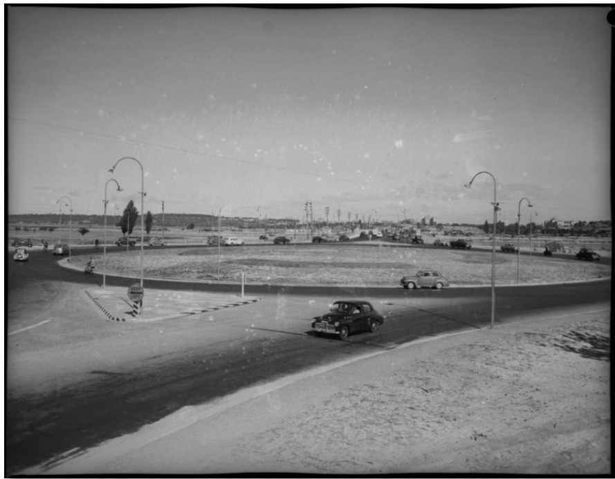
Figure 34. 1953 Roundabout at Victoria Park end of the Causeway (slwa_b3416445_2)
