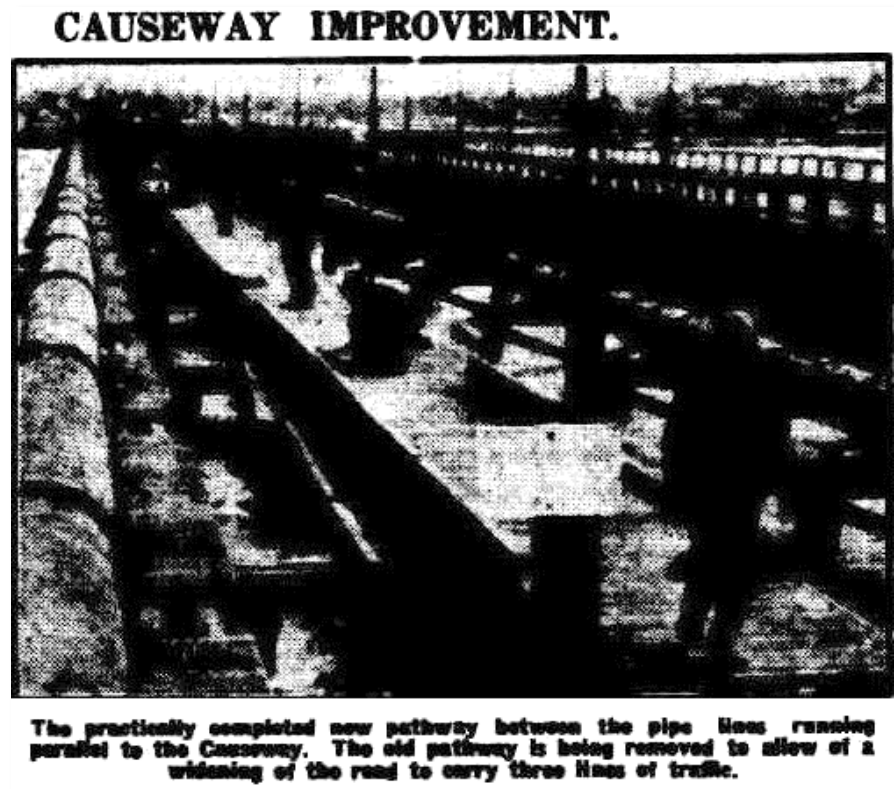
Figure 23. 1932 new pathway completed over the existing pipe trestles 38
