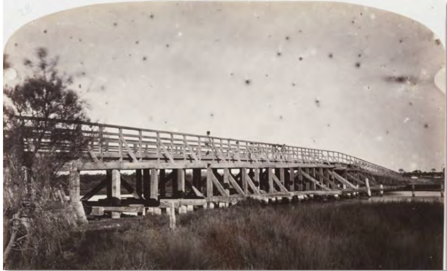
Figure 12. c.1865 North side of Causeway Bridge II (slwa_b3981178_1)
