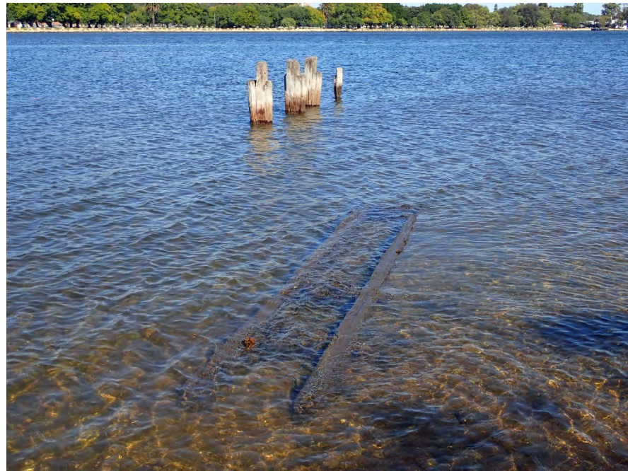
Plate 4. View southwest with pylon footings in foreground and timber piles in background
