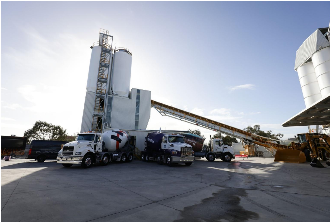
Figure 7: Covered conveyors at Holcim's Footscray Plant
