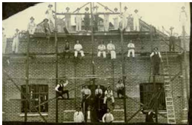
PH00005-05 Construction of the Bickford Soldiers Memorial Hall Source: Historypin.org
