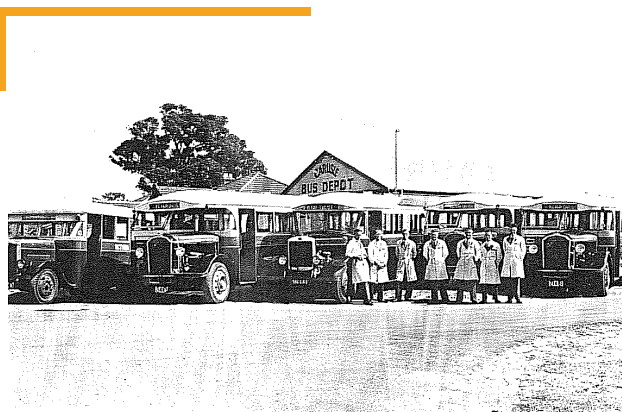
Photograph 35: The Carlisle Bus Depot before the MTT took over, c1958 (courtesy Geoff Gallop).
